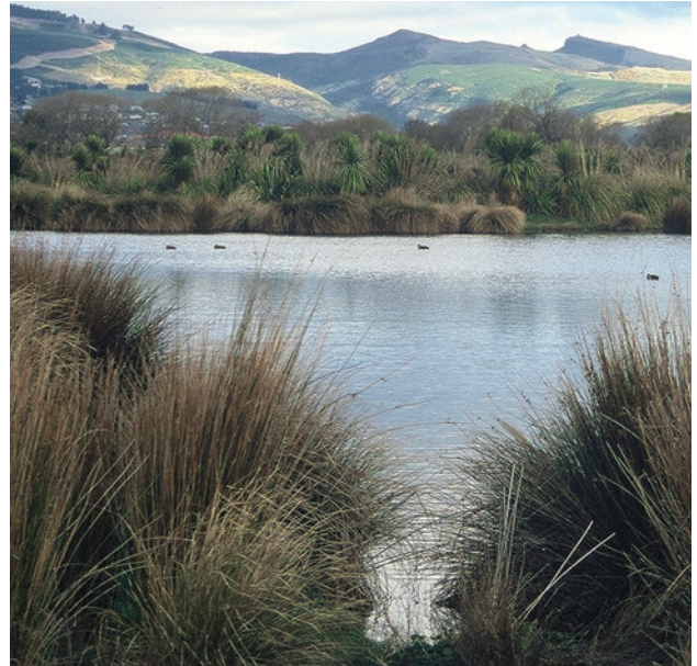
Figure 6-20: Wigram Detention Basin is a 3.5 ha flow-through wet pond that treats water from a 350 ha catchment in the Hornby district. Its large size and the surrounding reserve area has enabled the creation of a treatment facility with significant additional values.
