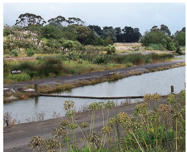
Figure 6-23: The pond and FWS wetland system at the Fletcher Building Steel Group industrial site, Auckland. Stormwater enters the pond from the bottom left, flows around the end of the “U” shaped system (centre right) and passes through the wetland, exiting at the left.
