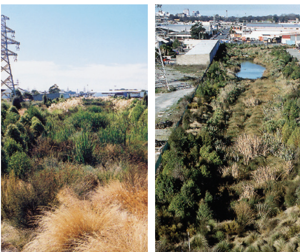
Figure 6-22: The Tranz Link constructed wetland system. Stormwater enters the intermittent free water surface (IFWS) wetland at the bottom of the photos and then enters two wet ponds, the first of which is visible at the top of the right photo.
