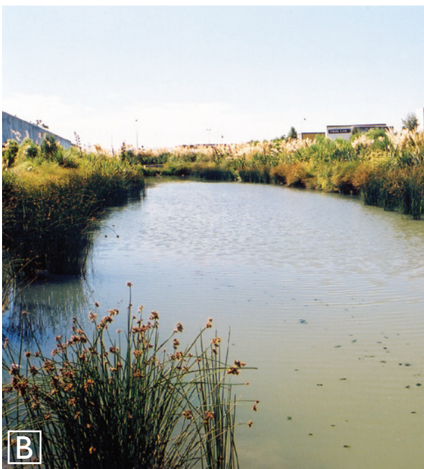
Figure 6-16A: Detention basins that are completely dry between rainfall events are called dry basins. They can be grassed or vegetated (as pictured here at Wrights Road).
