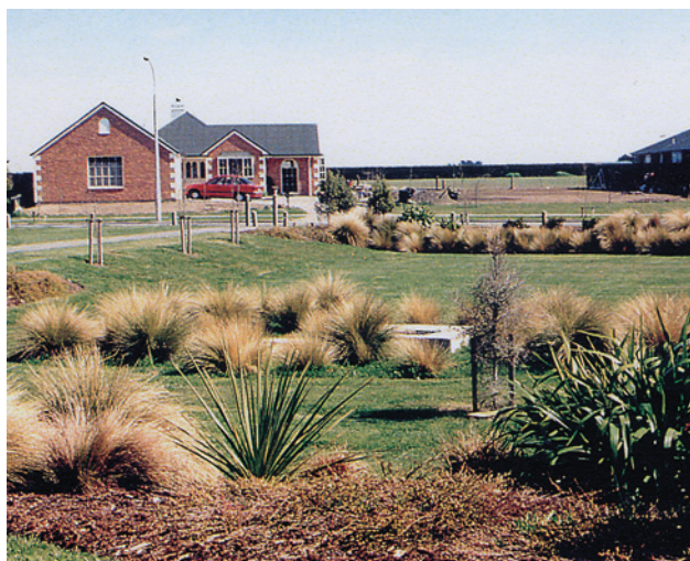
Figure 6-8: Soakage basins retain stormwater and allow soakage of stormwater through a filter bed, which removes contaminants. If appropriately designed, planted and placed in a reserve they can become a pleasing landscape element. Soakage basin in a local park along Roydon Drive.
