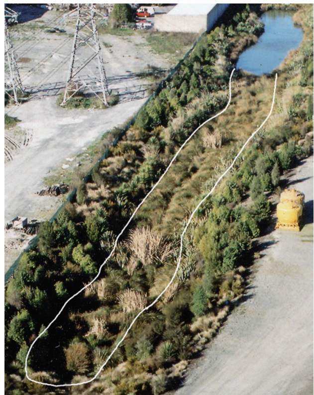
Figure 6-27: Constructed wetlands should have a length:width ratio of 10 L:1W to simulate plug flow. Tranz Link wetland, Matipo Street. The white line represents the wetland base area.
