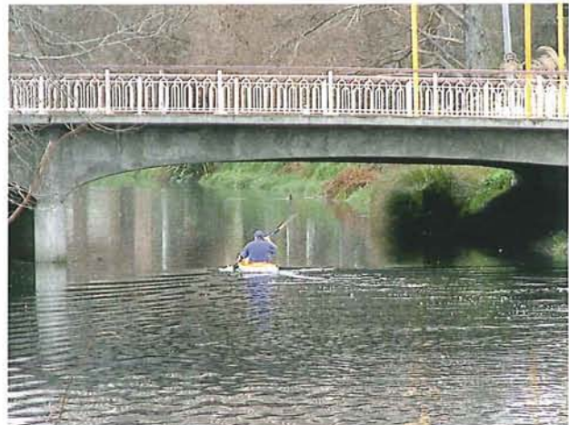
Figure 13-9: For non-tidal rivers with boat passage, bridge soffit level must exceed mean flow water level plus one meter freeboard. Avon River/Ōtākaroro at Stanmore Road.
