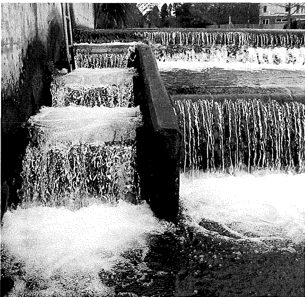
Figure 13-12: Two fish ladders have been installed on each side of the Mona Vale weir to facilitate the upstream passage of trout. Note that designing for trout passage may not provide for the passage of native fish.
