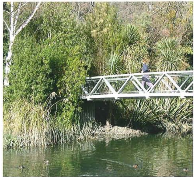
Figure 13-5: Planting around a bridge headwall will help to screen any heavy engineering structures. Heathcote River/Ōpāwaho footbridge at Aynsley Terrace, Hansens Park.
